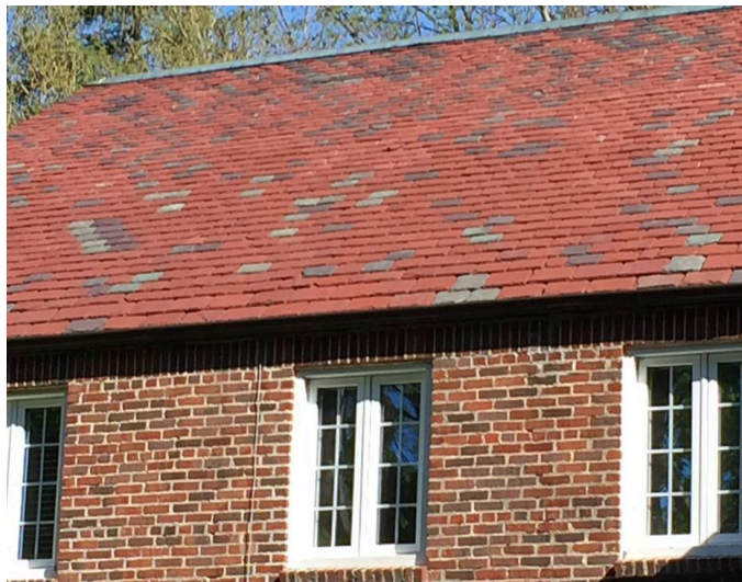
Figure 5: Second-story windows and the red and gray slate, cross-hipped roof.
