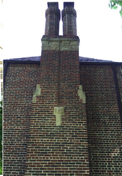
Figure 4: More stone accents can be found on the left side of the house, which features a large, double shaft chimney capped with two octagonal chimney pots. Note the English Bond brick pattern to the right of the chimney and the American cross bond brick pattern not only on the chimney but also to the left.
