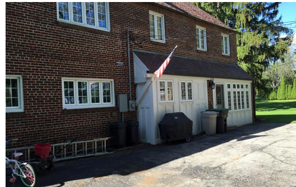
Figure 6: On the right side of the house, along the driveway, a garage has been converted into a second family room, which reveals itself by its white board-and-batten siding and steeply pitched shed roof.
