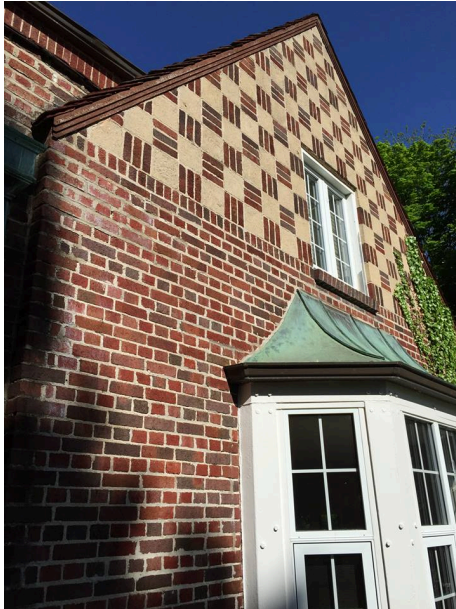
Figure 2: The dominant feature of the home is a prominent checkerboard pattern of red bricks and tan stucco in the gable—with the bay window located below.
