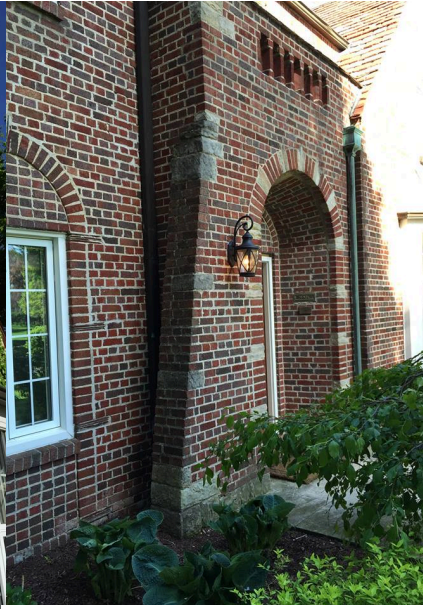
Figure 3: The architects created emphasis around the home's entrance through the addition of a few stone accents. Note the sloping, "battered" wall to the left of the entrance.
