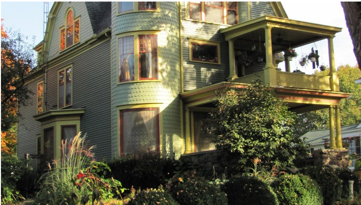
View from the northwest corner showing the variety of surface materials, the Palladian window, the bay window, and the rebuilt double-decker porch with Ionic and Tuscan columns. Photograph by Amy Garno, 2010.
