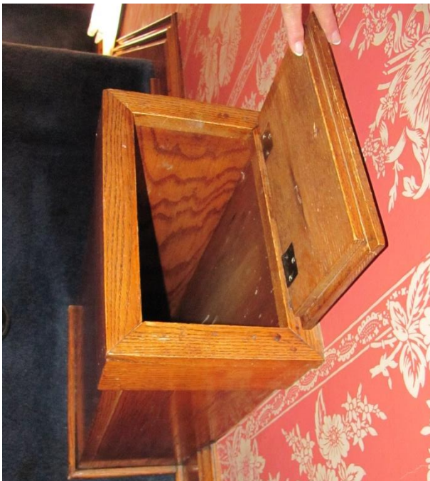
The laundry shoot in the second story hallway leads down to the kitchen, below. Photograph by Amy Garno, 2010.
