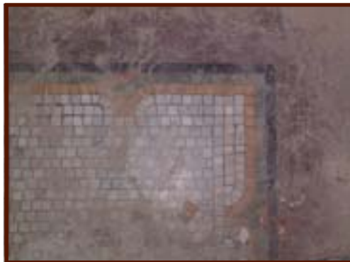
Detail photo of original terrazzo floor before being covered.
